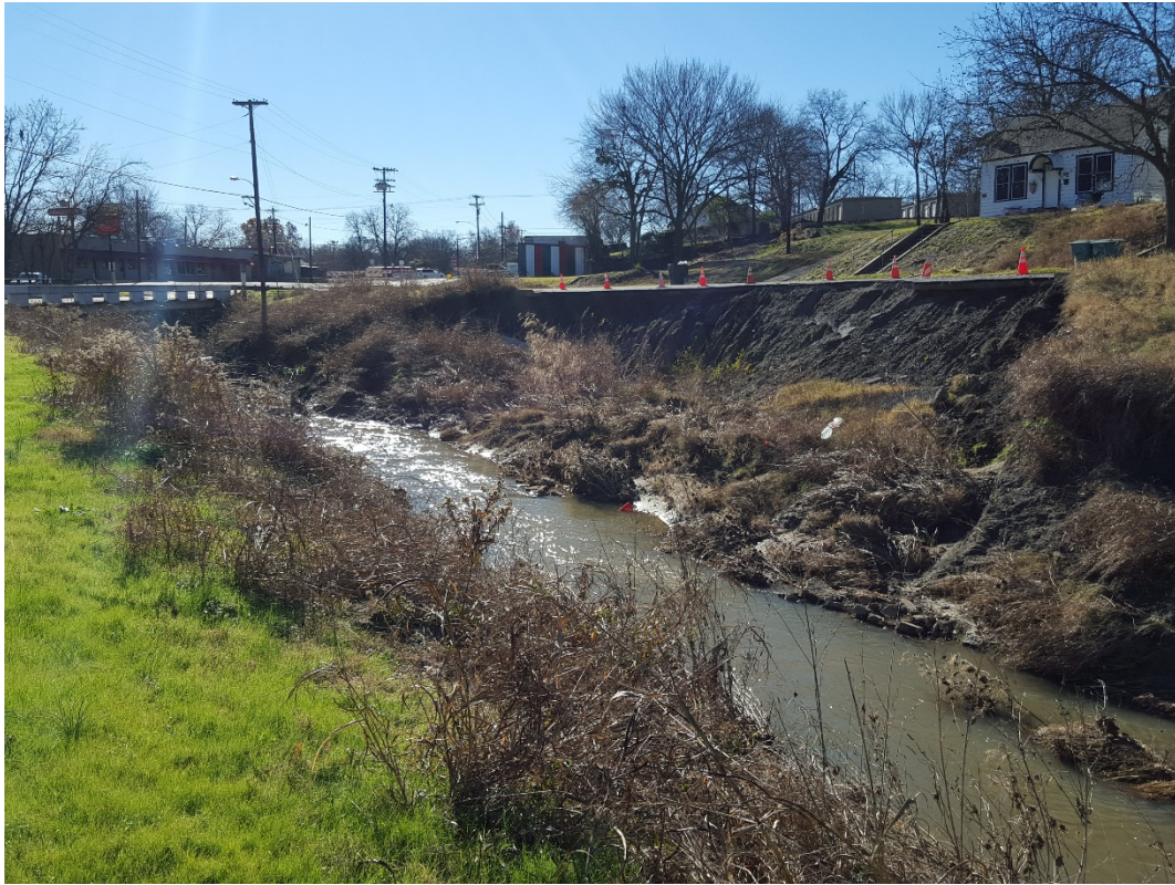
Kessler Blvd. Looking South from East Side of Creek
