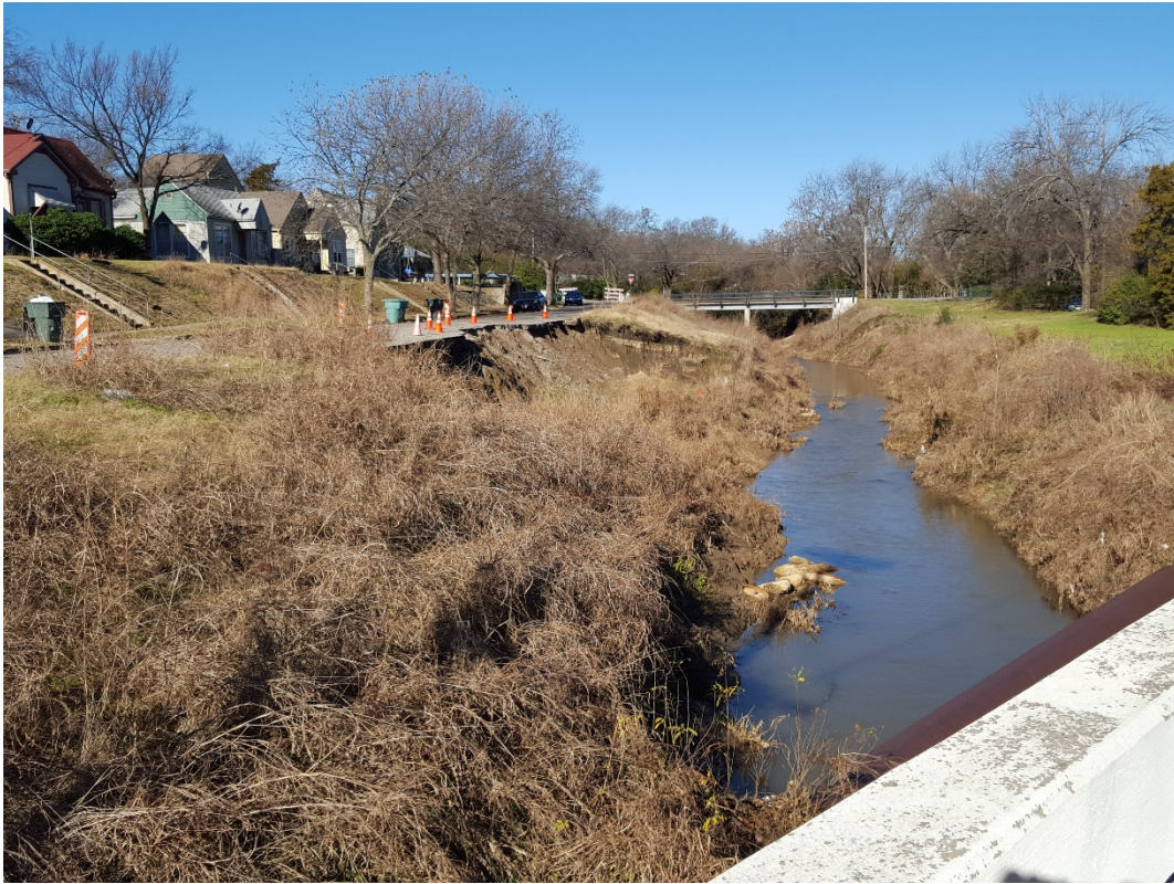
Kessler Blvd. Looking Northwest from Woods St. Bridge
