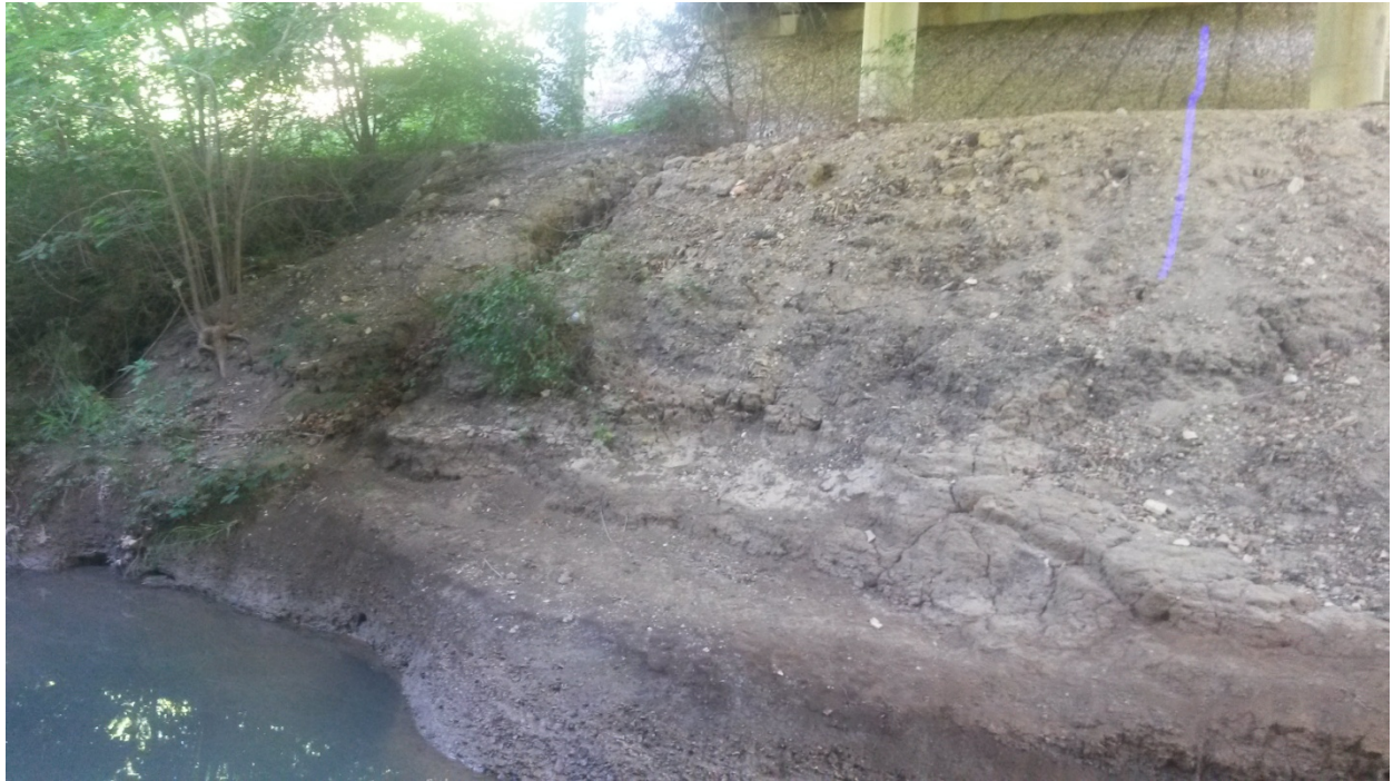
Fallon Drive Bridge – West Embankment
