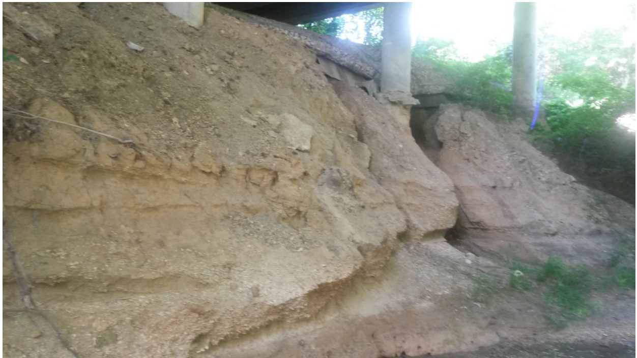
Fallon Drive Bridge – East Embankment
