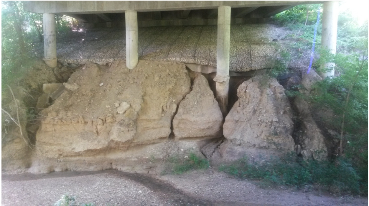
Fallon Drive Bridge – East Embankment
