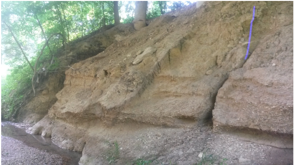
Fallon Drive Bridge – East Embankment
