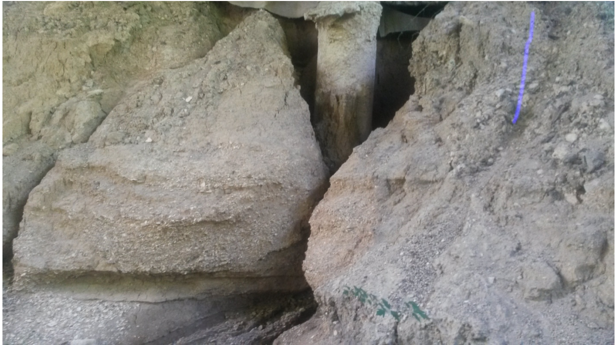
Fallon Drive Bridge – East Embankment
