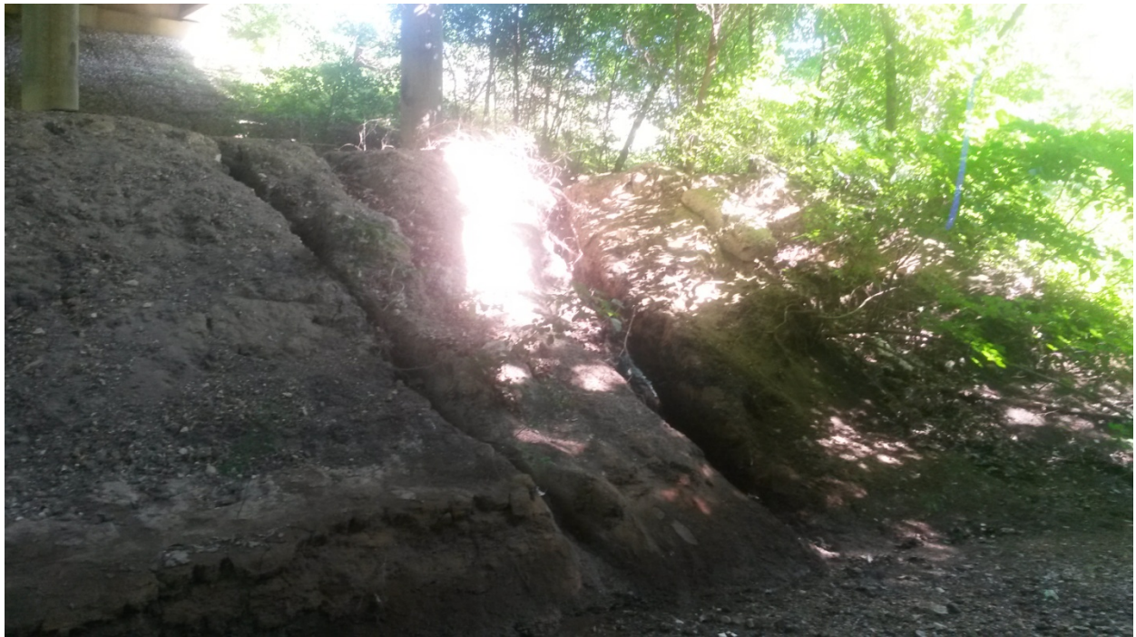
Fallon Drive Bridge – West Embankment
