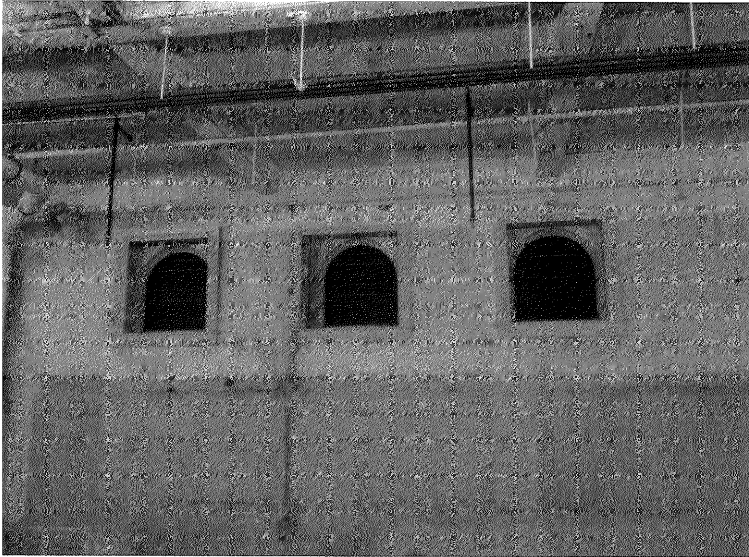
Arched red glass windows which will be restored and remain in the completed project. These windows are visible in the first historic photo taken approximately 1876.
