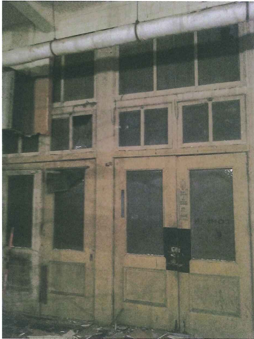
Doors on south side of building. It is proposed these be incorporated into the historic interior design.
