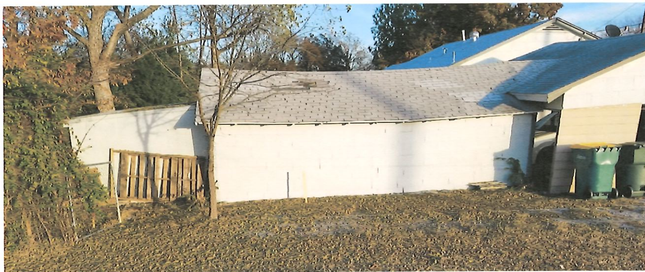
West side of original garage in between a shed and the carport.
