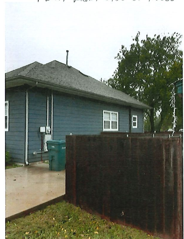
FRONT RIGHT SIDE OF HOUSE
