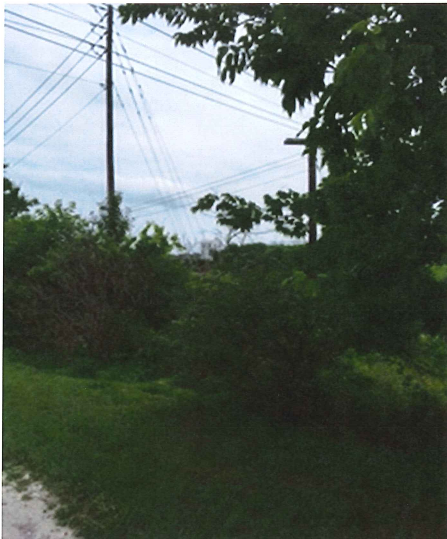
View of Southern neighbor TXU Sub Station property
