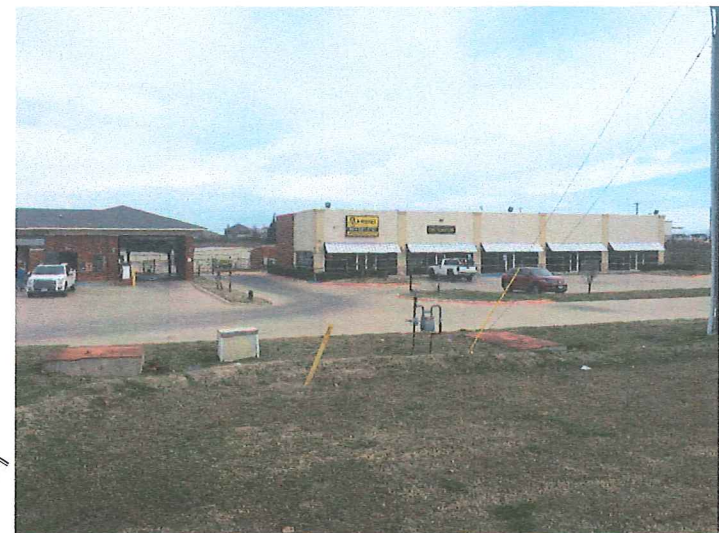
WEST ELEVATION OF THE EXISTING RETAIL BUILDING
