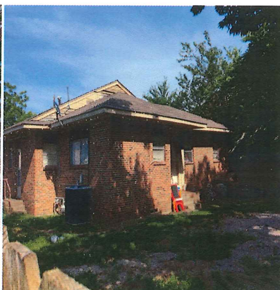
Back view facing West
