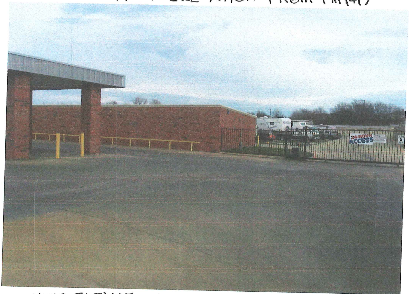
WEST ELEVATION PAST CARWASH & RETAIL BUILDING
