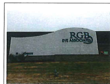
EXISTING SIGNAGE - TO BE REMOVED
