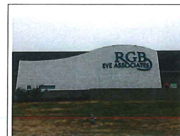
EXISTING SIGNAGE - TO BE REMOVED
