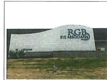
EXISTING SIGNAGE - TO BE REMOVED
