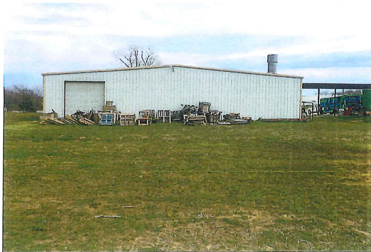
Existing building on Subject Property Back
