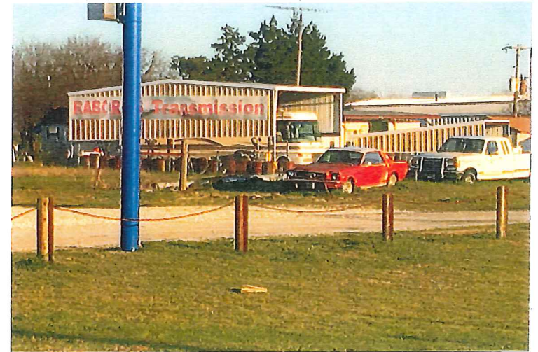
Building facing Mission Dr. west side
