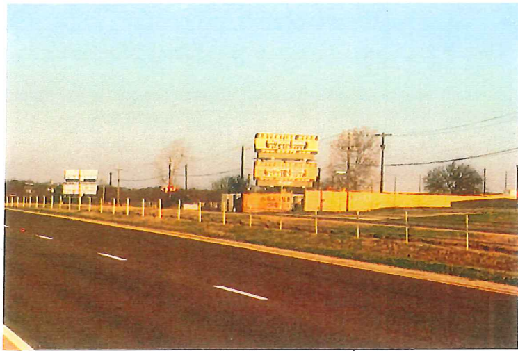
Adjacent buildings on Hwy 82
