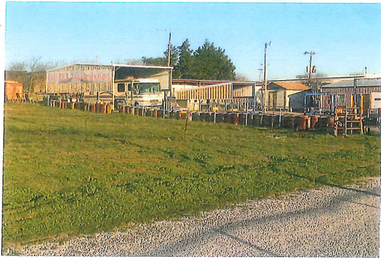
Building facing Mission Dr West side
