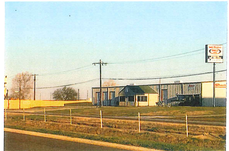
Adjacent buildings on Hwy 82
