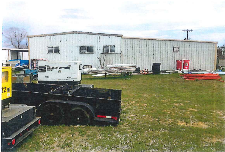
Existing Building on Subject Property Back
