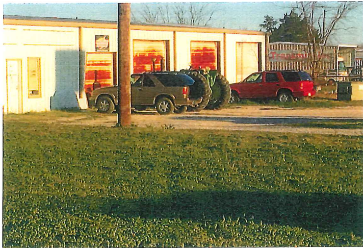
Building facing Mission Dr. West side.
