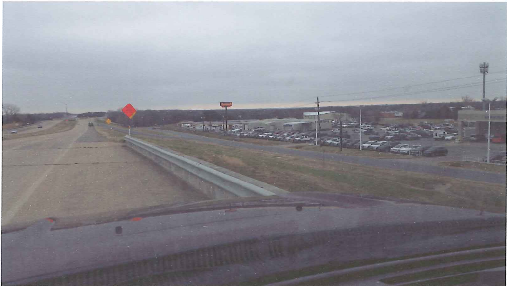
US HWY 82 - OVERPASS BRIDGE
