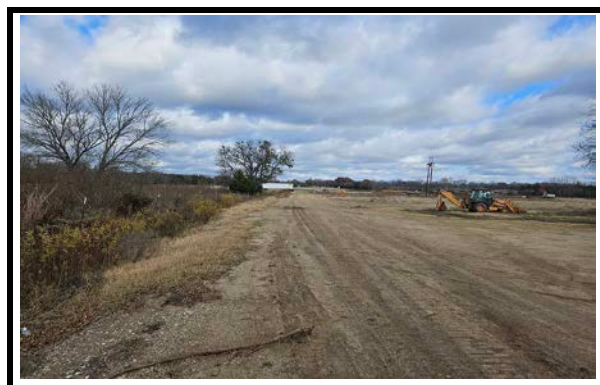
DIRT ROAD ACCESS FROM NORTH
