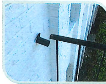
Unsafe Handrail
