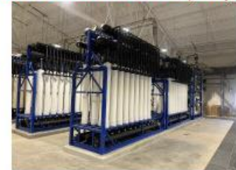
Added 5-MGD UF/RO Capacity
