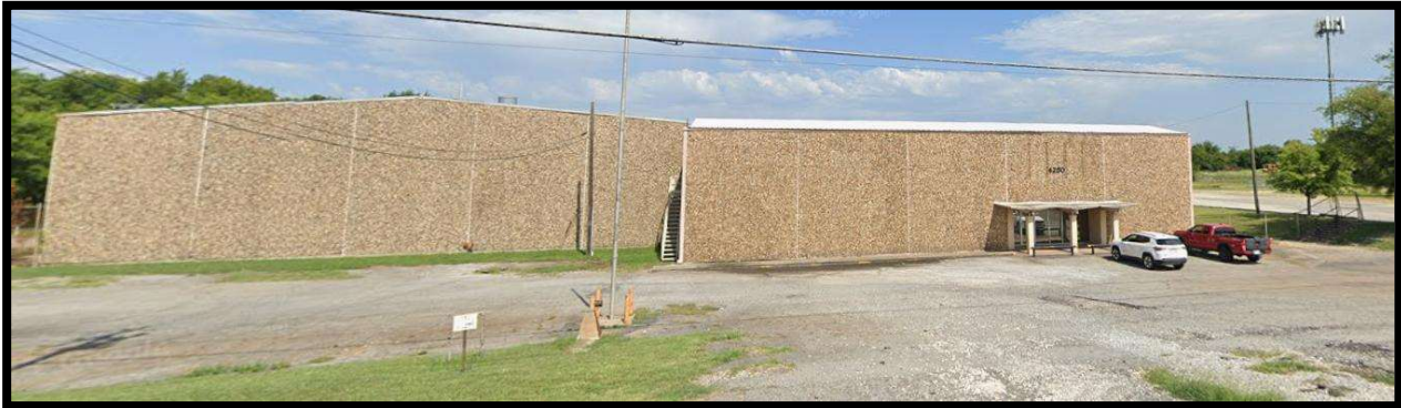
Front of the building before:
