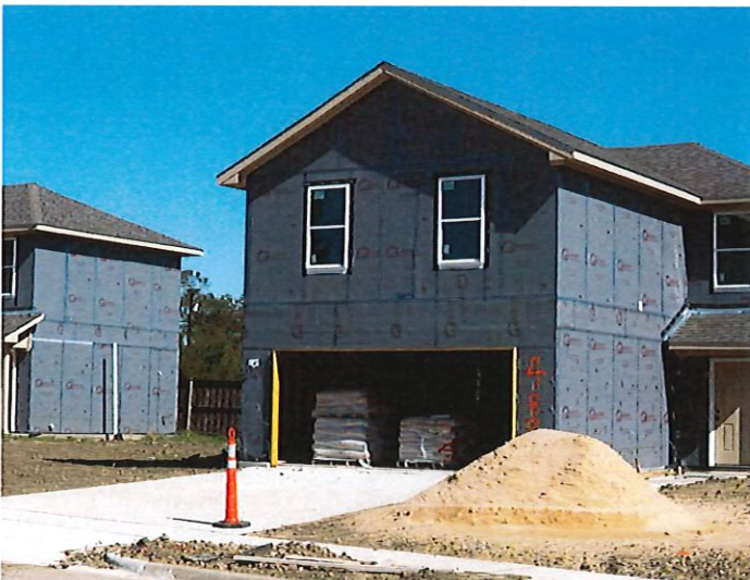
New housing development in Sherman
