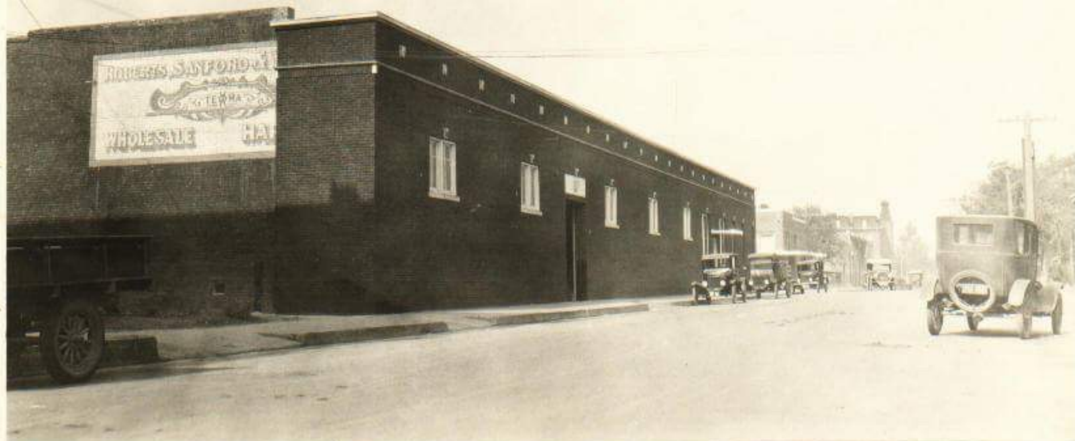
Valmont St. front 193 1/2' showing front entrance with this door.
