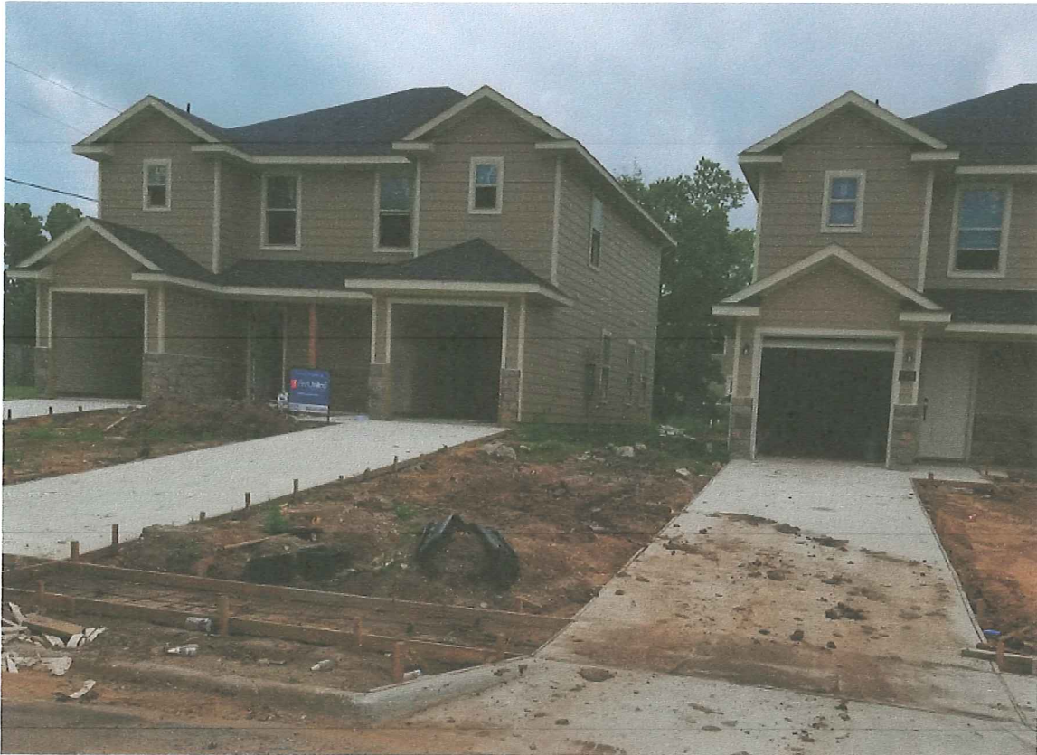
New Construction – Forest & S Crockett
