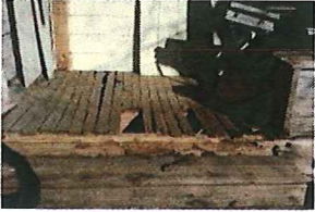
ont porch flooring.20160113_0
