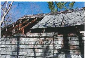
roof. west side.20160328_144
