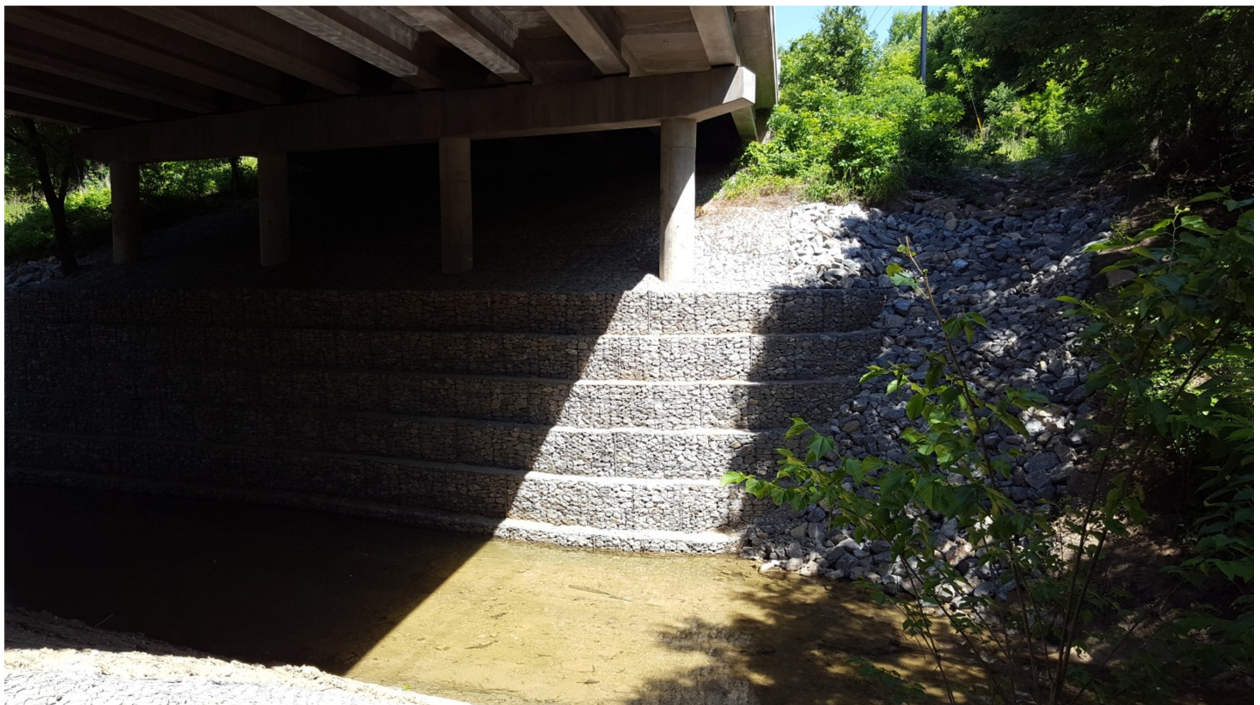
Fallon Bridge Erosion Control – After
