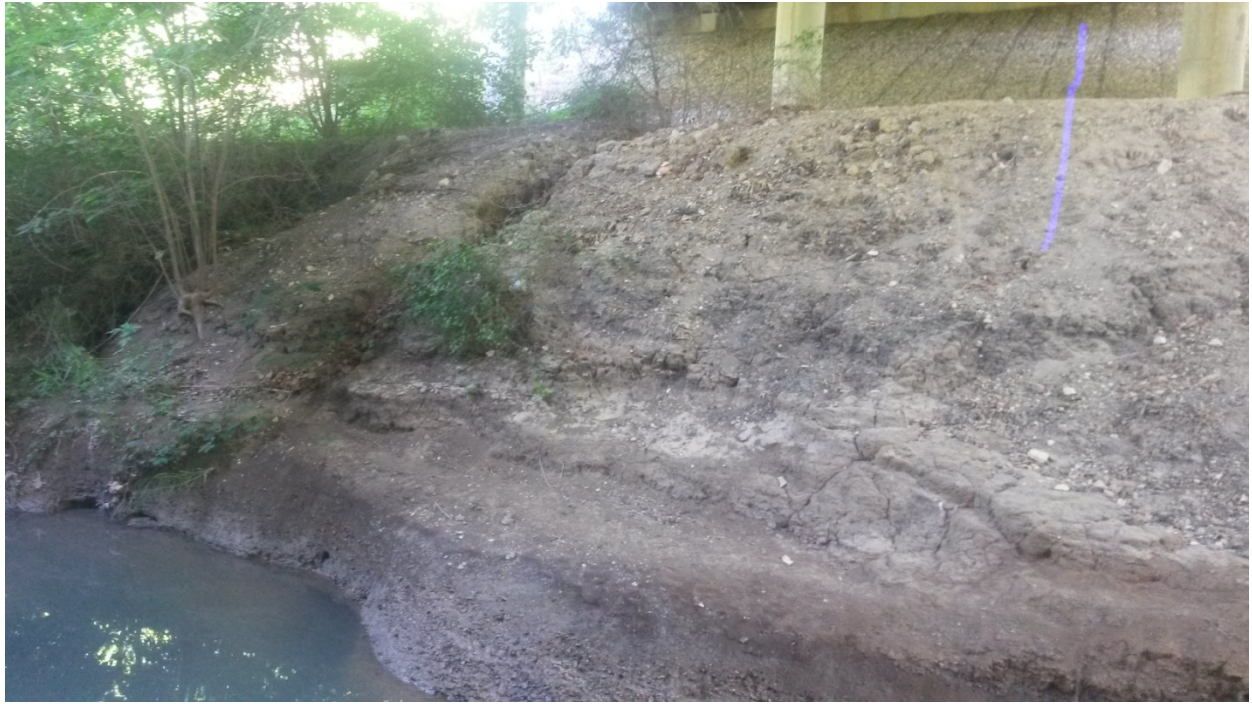
Fallon Drive Bridge – West Embankment
