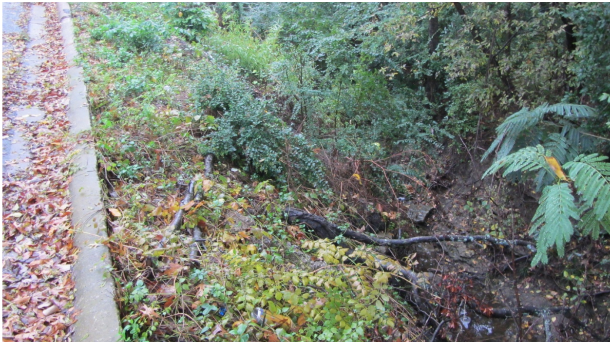
Hunt Street – From edge of roadway looking down
