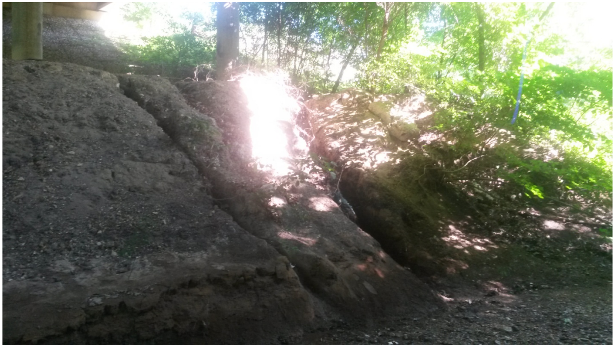
Fallon Drive Bridge – West Embankment
