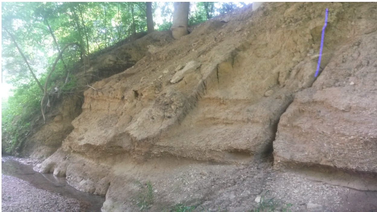
Fallon Drive Bridge – East Embankment
