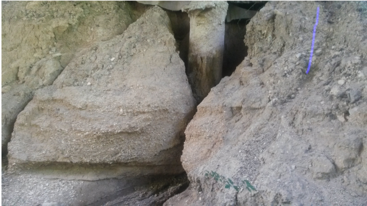
Fallon Drive Bridge – East Embankment
