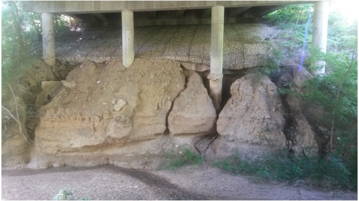
Fallon Drive Bridge – East Embankment
