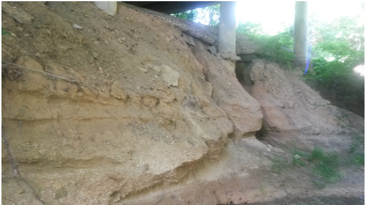
Fallon Drive Bridge – East Embankment
