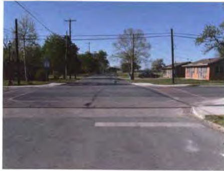
Intersection of Brockett and Willow looking north
