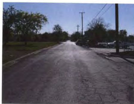
Intersection of Pacific and Porter looking west
