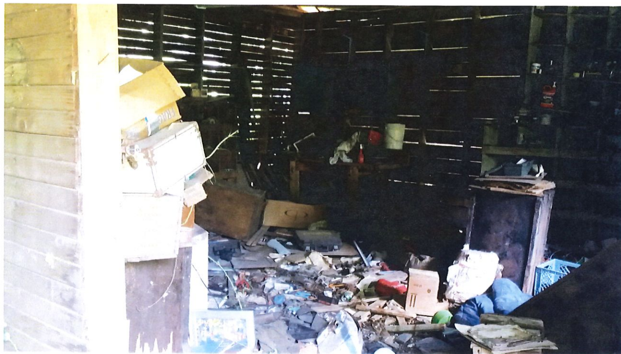
Rear unsecured building:
