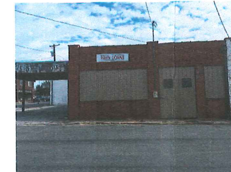
WEST ELEVATION FROM ELM ST.
